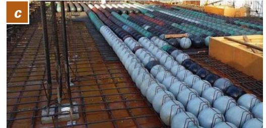
Figure 1 – Void formers (a) BubbleDeck® – Semi-precast system (b) BubbleDeck® – Cast-in-place system (c) Cobiax USA® – Cast-in-place system (Photos courtesy of BubbleDeck and Cobiax USA).
