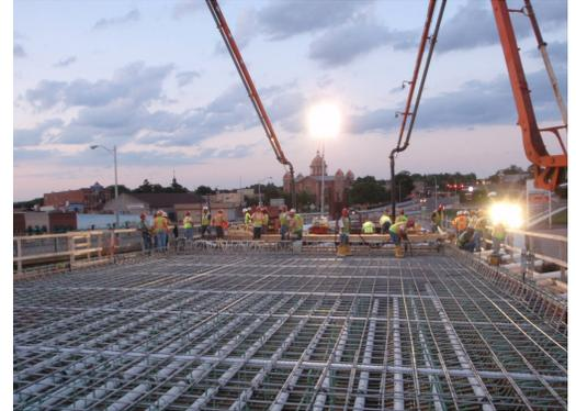
Figure 1 – Stainless steel reinforcing bar used in the deck of a bridge structure located in Minnesota.
